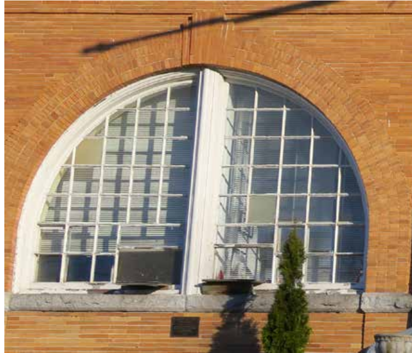
Existing painted wood windows with single glazing
