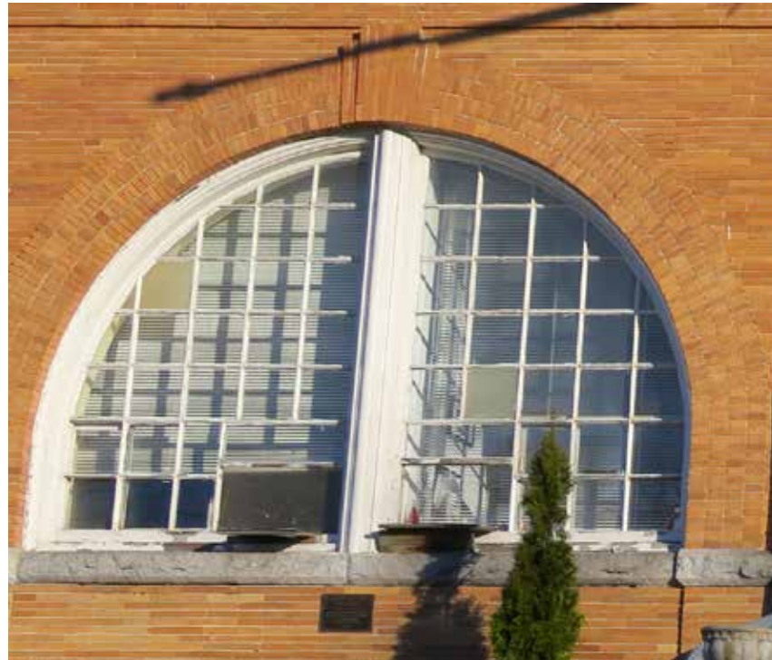
Existing painted wood windows with single glazing
