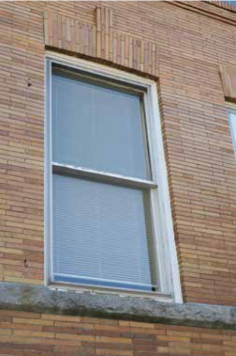
Existing painted wood windows with single glazing
