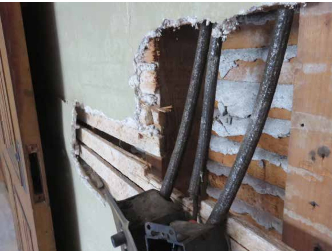
Existing wood studs with lath and plaster
