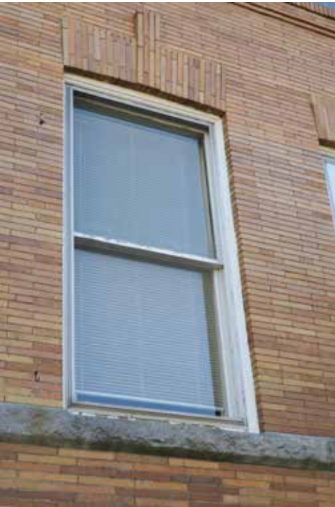
Existing painted wood windows with single glazing
