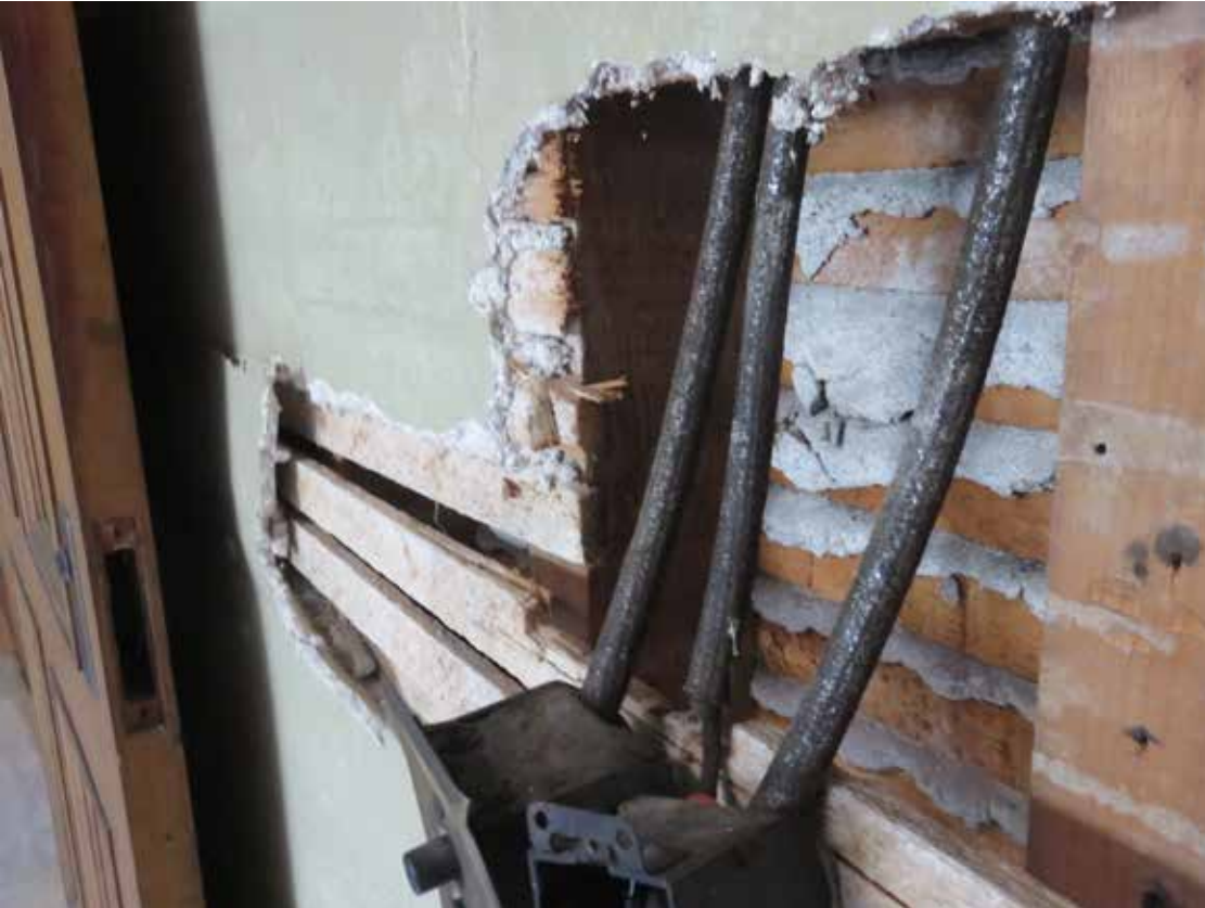
Existing wood studs with lath and plaster
